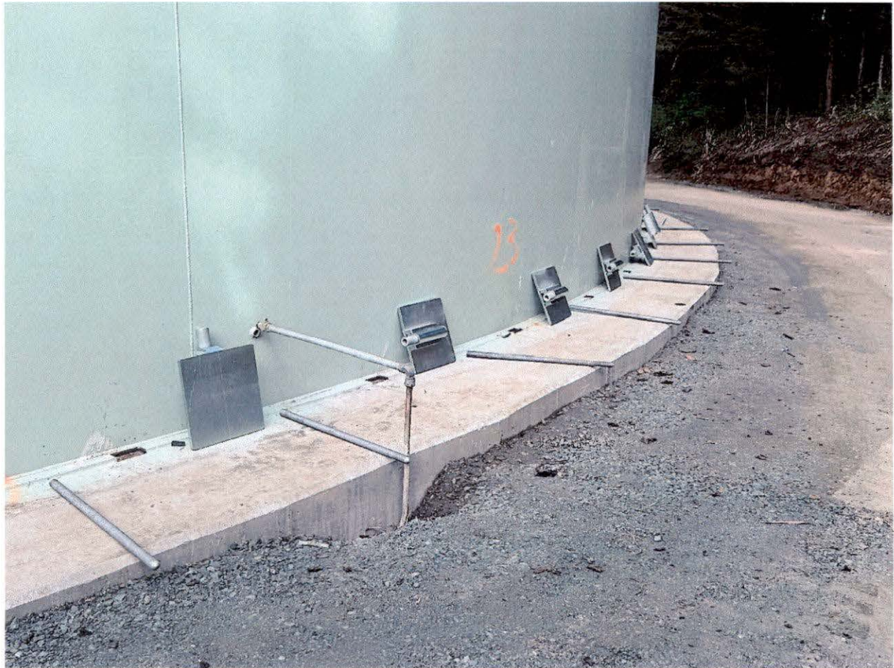
April 15, 2026 – Preping for anchor chair installation.
