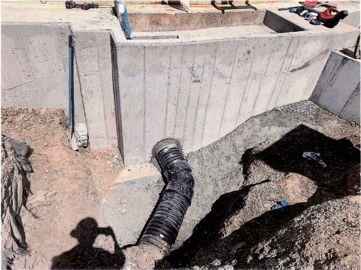
April 8, 2026 – View of new drainage basin at overflow/flush cleanout.
