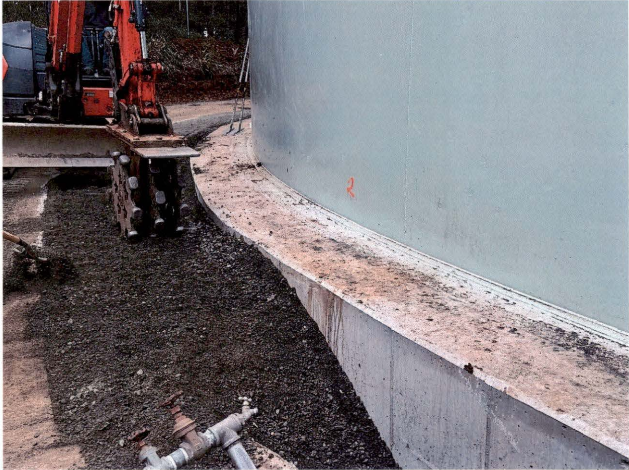
April 6, 2026 – Backfilling against the foundation.
