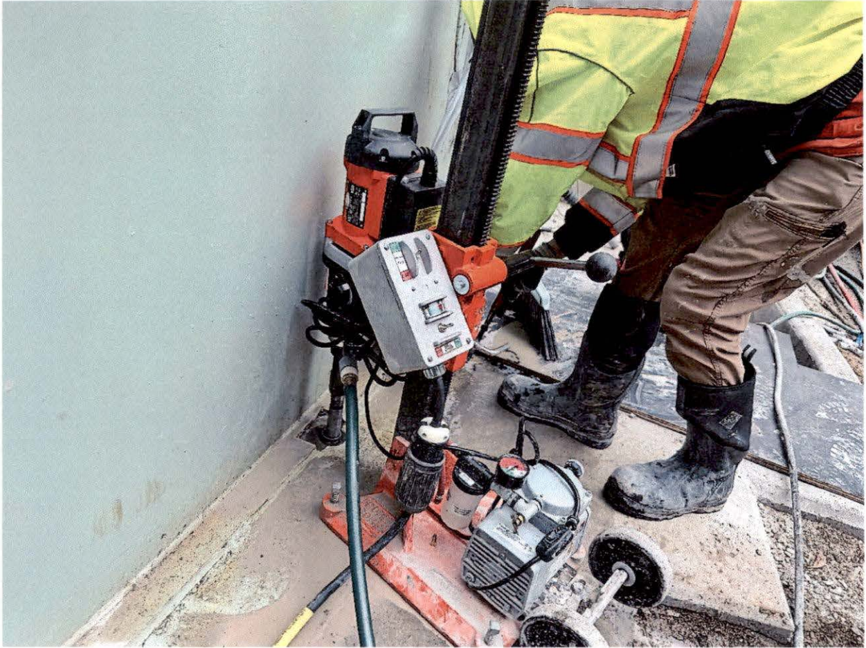
April 29, 2026 – Core drilling to accommodate new anchor chairs.
